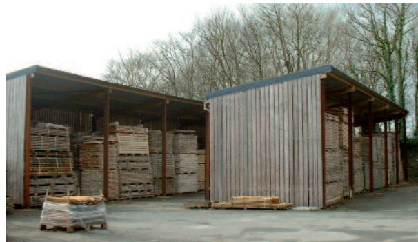
The use of locally produced low-impact materials and new techniques may produce appropriate contemporary buildings (Coed Cymru wood store, Pembrokeshire)
