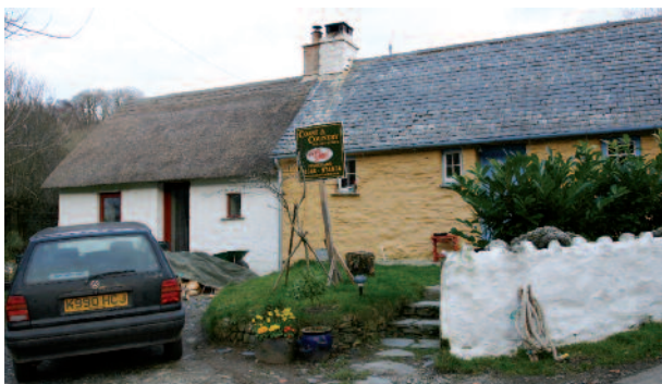
Re-use of existing building combined with use of traditional clom walled and thatch roof extension
