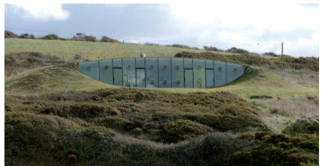
Scale, mass and form must be carefully judged whether designing in settlements or projects in the landscape
