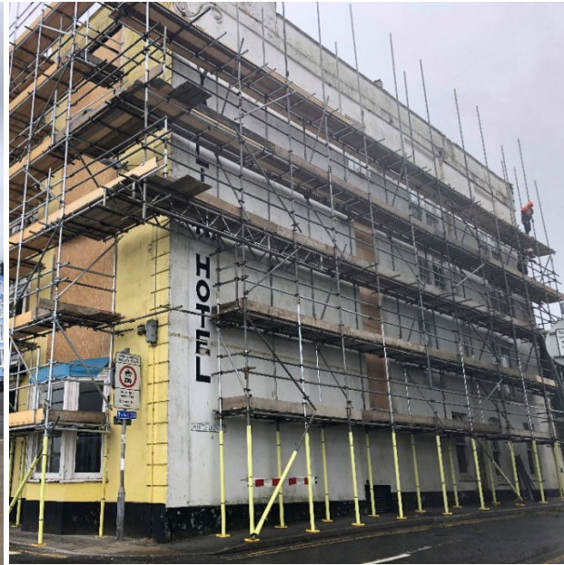
Works underway at Royal Lion Hotel 2024
