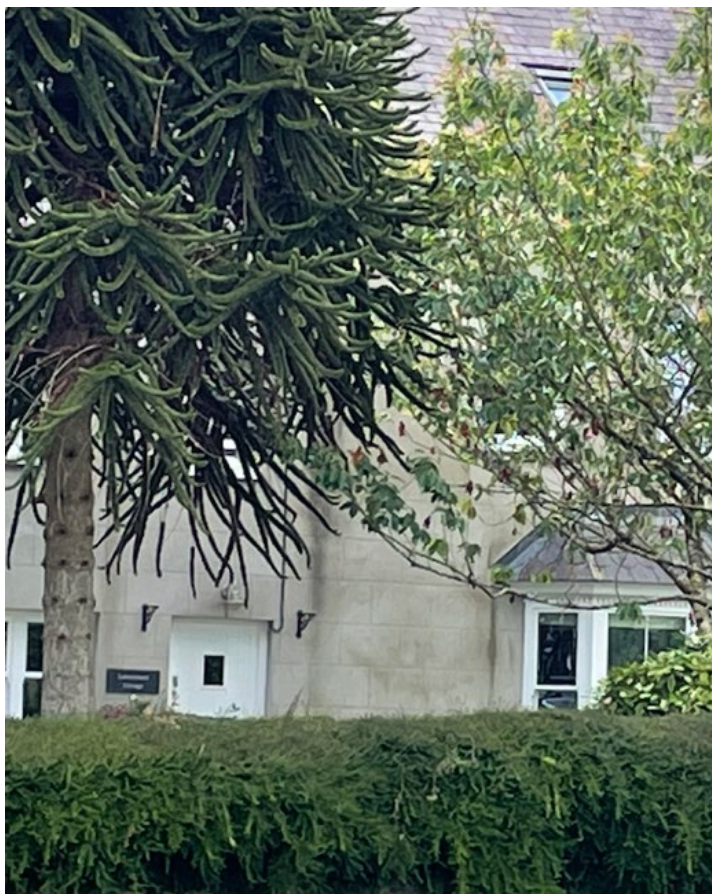
Figure 8: Photograph showing a building with scribed render
