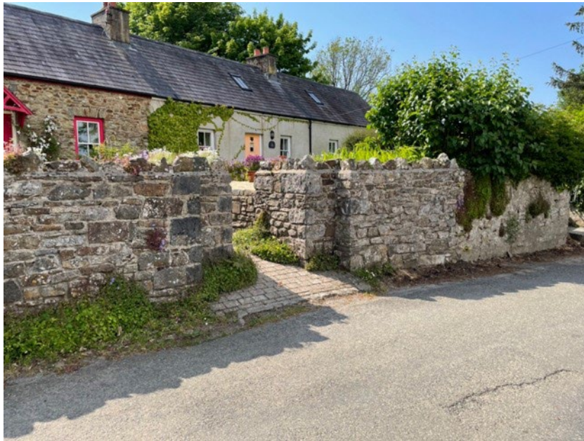
Figure 22: Photograph showing stone boundary wall with a cock and hen top.
