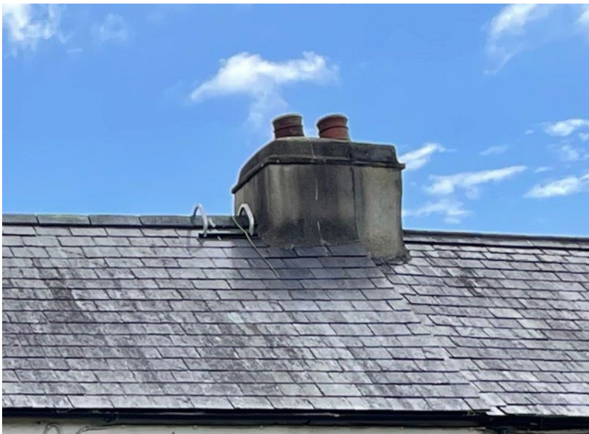
Figure 19: Photograph showing a smooth rendered chimney
