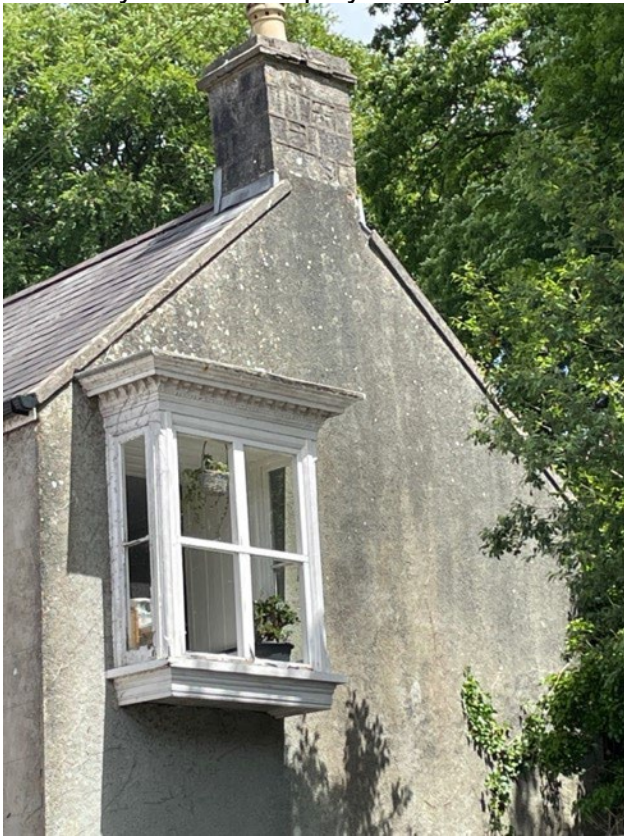
Figure 13: Photograph showing a cantilevered rectangular bay window
