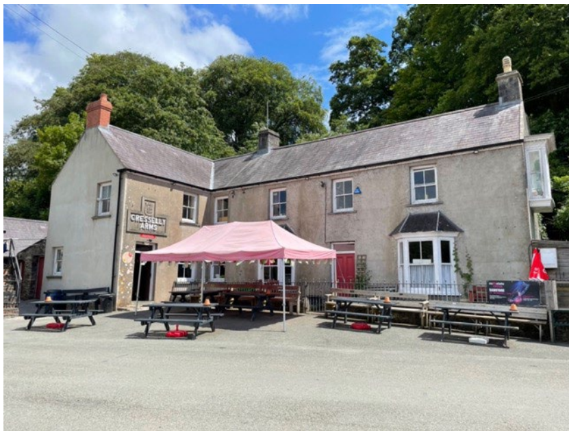
Figure 17: Photograph showing gabled and slated roof
