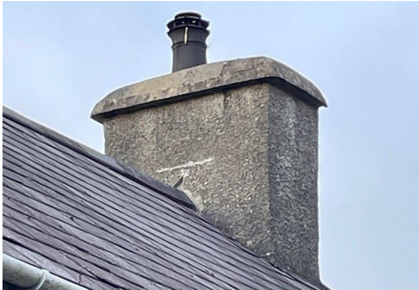
Figure 20: Photograph showing a roughcast rendered chimney.
