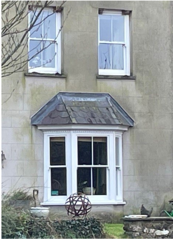
Figure 14: Photograph showing a splayed bay window
