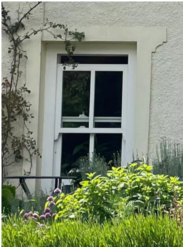
Figure 11: Photograph showing a 4 paned sash window with horn details
