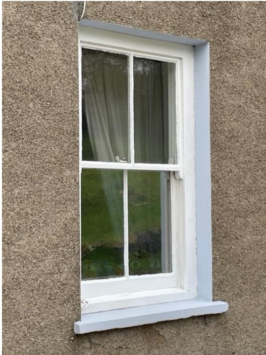
Figure 10: Photograph showing a 4 pane sash window
