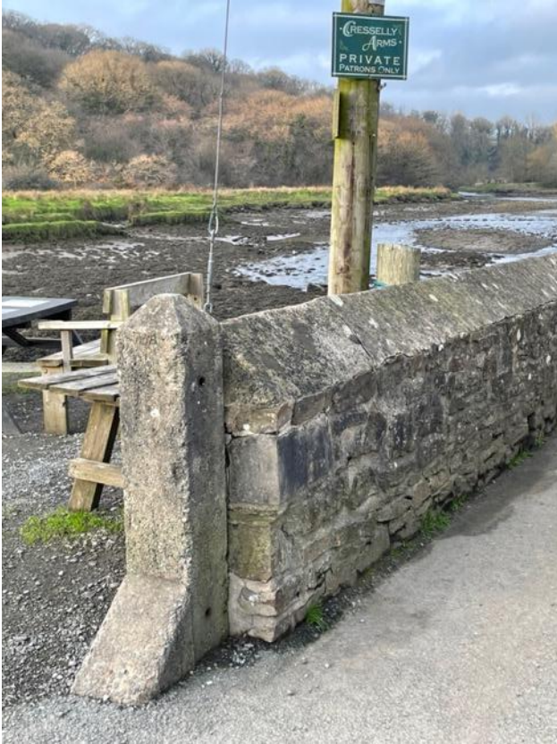
Figure 24: Photograph showing an example of sloping rendered copings to stone walls around the village.
