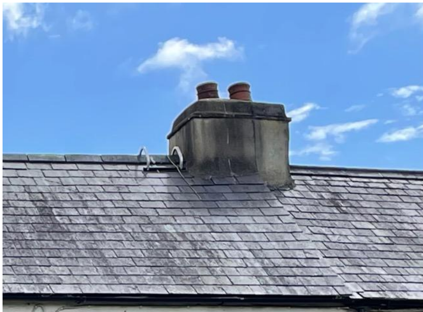
Figure 19: Photograph showing a smooth rendered chimney
