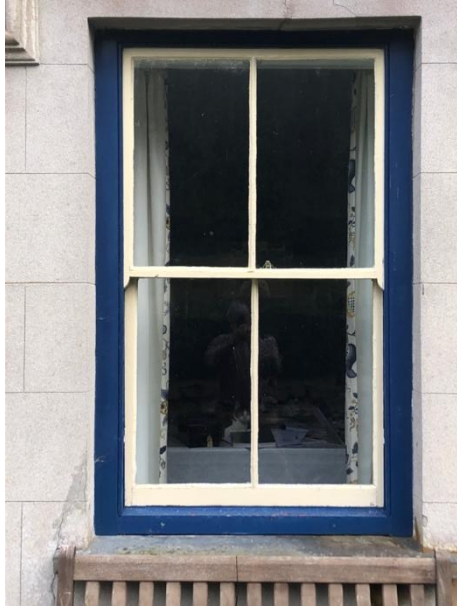
Figure 39: Photograph showing blue painted outer lining of sash window.
