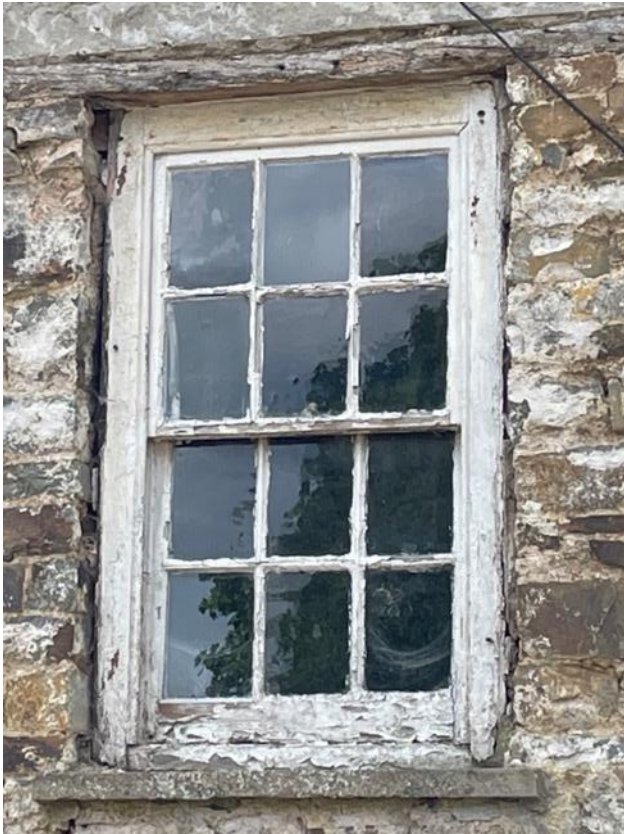
Figure 12: Photograph showing a 12 pane sash window
