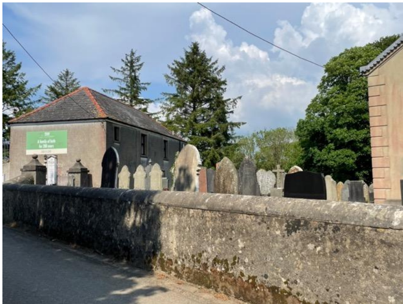
Figure 23: Photograph showing curved rendered copings to stone walls in the village.
