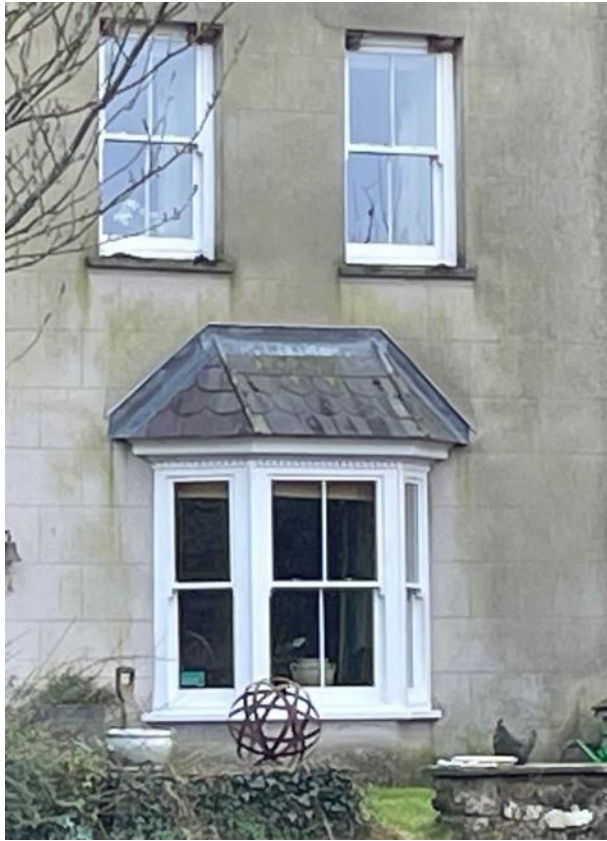
Figure 14: Photograph showing a splayed bay window
