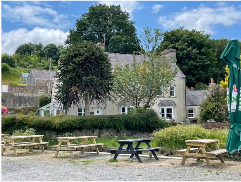
Figure 18: Photograph showing a group of buildings with pitched roofs with gabled ends.
