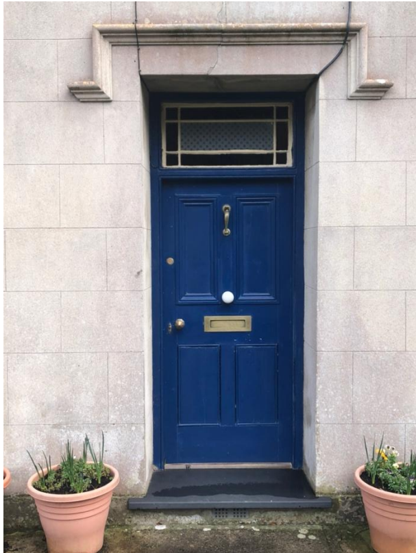
Figure 16: Photograph showing a panelled door with stained glass detailing above.
