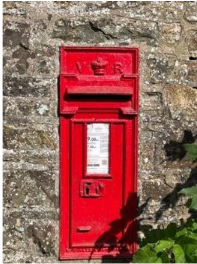
Figure 26: Photograph showing the red post box inset into a stone wall
