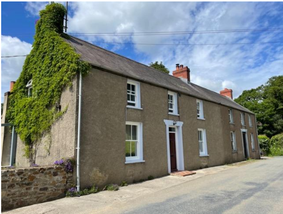
Figure 6: Photograph showing properties with unpainted render
