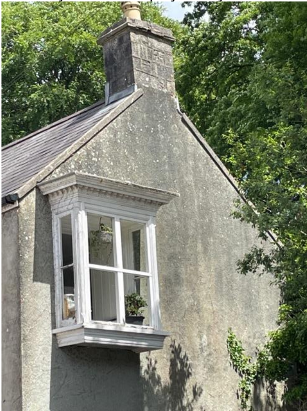
Figure 13: Photograph showing a cantilevered rectangular bay window
