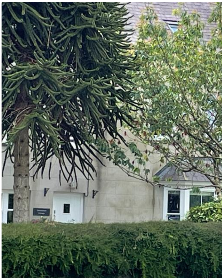
Figure 8: Photograph showing a building with scribed render
