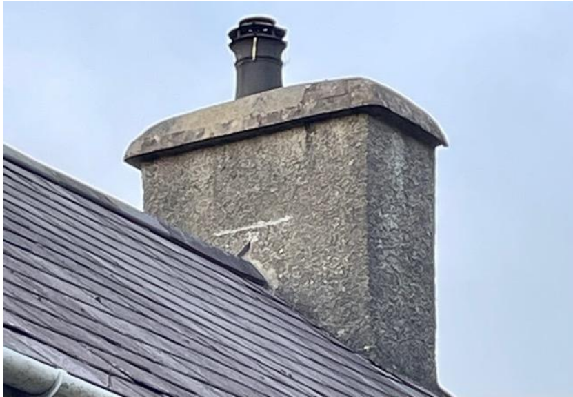
Figure 20: Photograph showing a roughcast rendered chimney.
