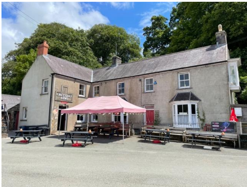
Figure 17: Photograph showing gabled and slated roof
