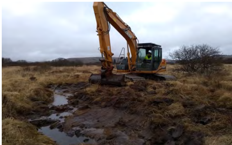
Modifying flushes to create Southern Damselfly habitat.
